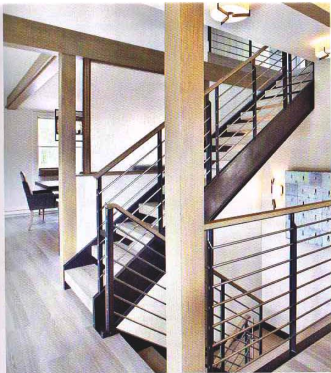
Designed by the architect Eric Cummings, the stairwell features a blend of rolled steel, with ash treads and oak bar details. The black and silver color variations are a result of using different steel materials with a clear lacquer finish.
